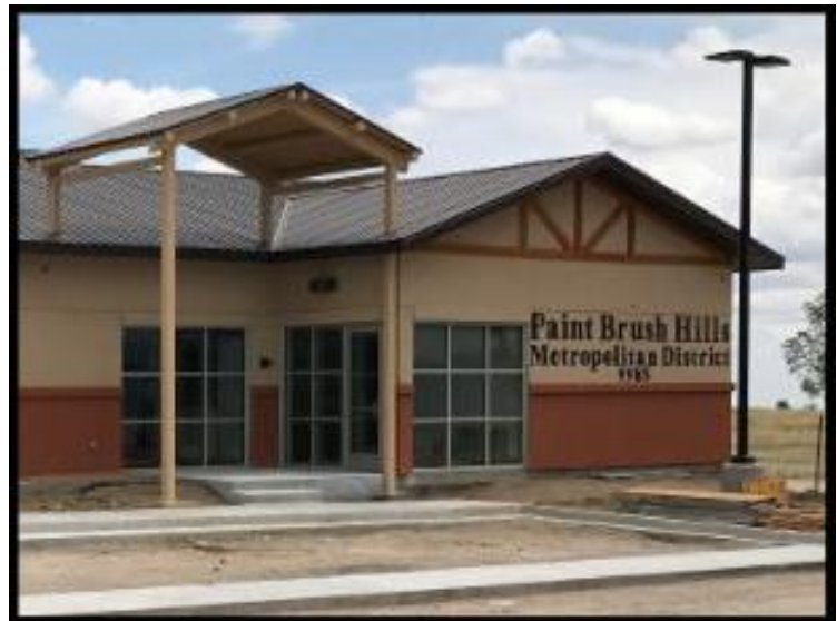
Maintenance area entry.
