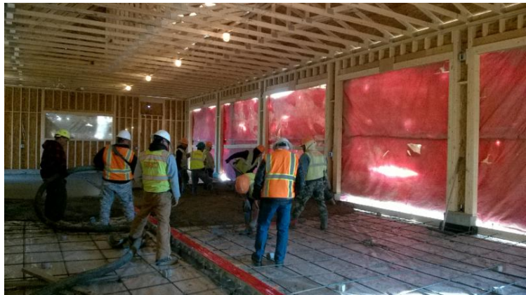
Concrete being layed on the maintenance area floor.
